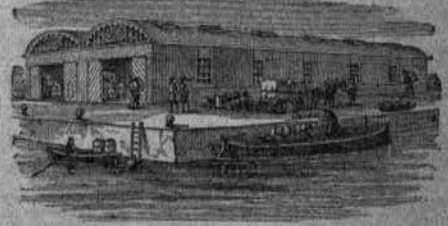
RAILWAY OR WHARF GOODS WAREHOUSE
