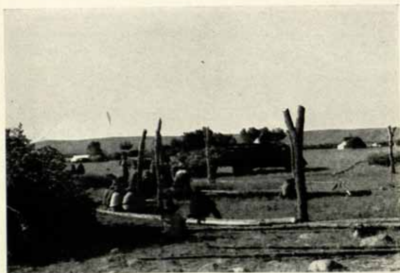
Upper: Measuring radii to locate side-post holes from the center pole. July 3, 1937. Lower: Compton, stooped over, fixing the buffalo head onto the center pole. Tassitsie, right, is painting it. Note the Indian Service truck used to haul branches.
