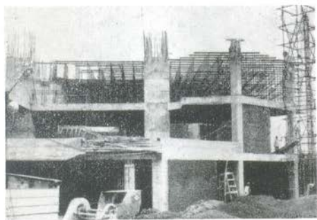
Construction under way at the Nehru Science Centre, Bombay
